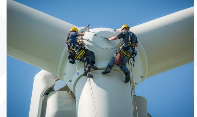
Challenge 3 – Operation & Maintenance and Digitalisation
